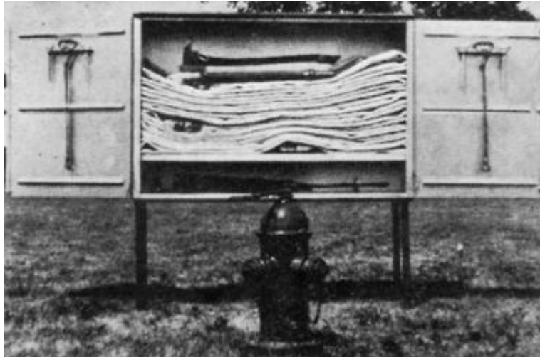
FIGURE A.3.3.14(c) Hose House That Can Be Installed on Legs, As Pictured, or on a Wall Near, but Not Directly over, a Private Hydrant.
